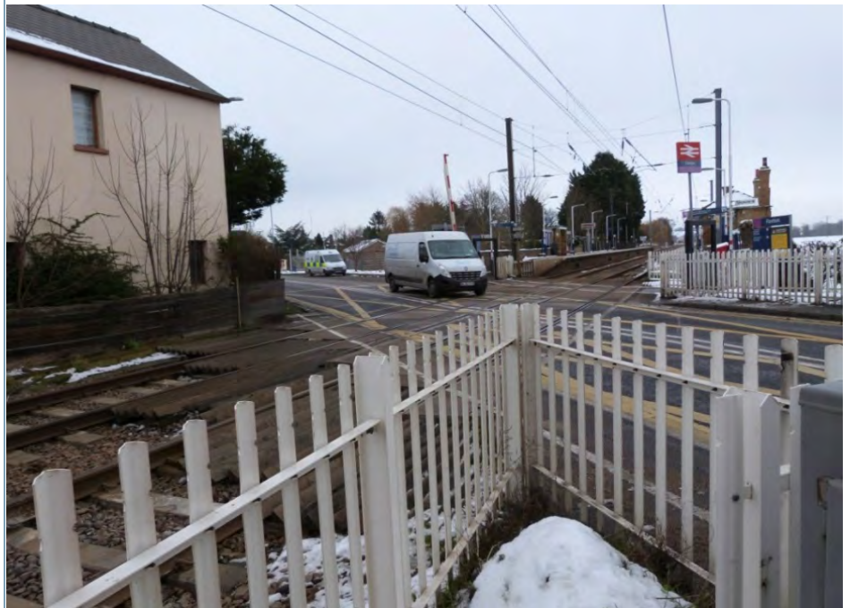
Photo 1.3: Existing Level Crossing
