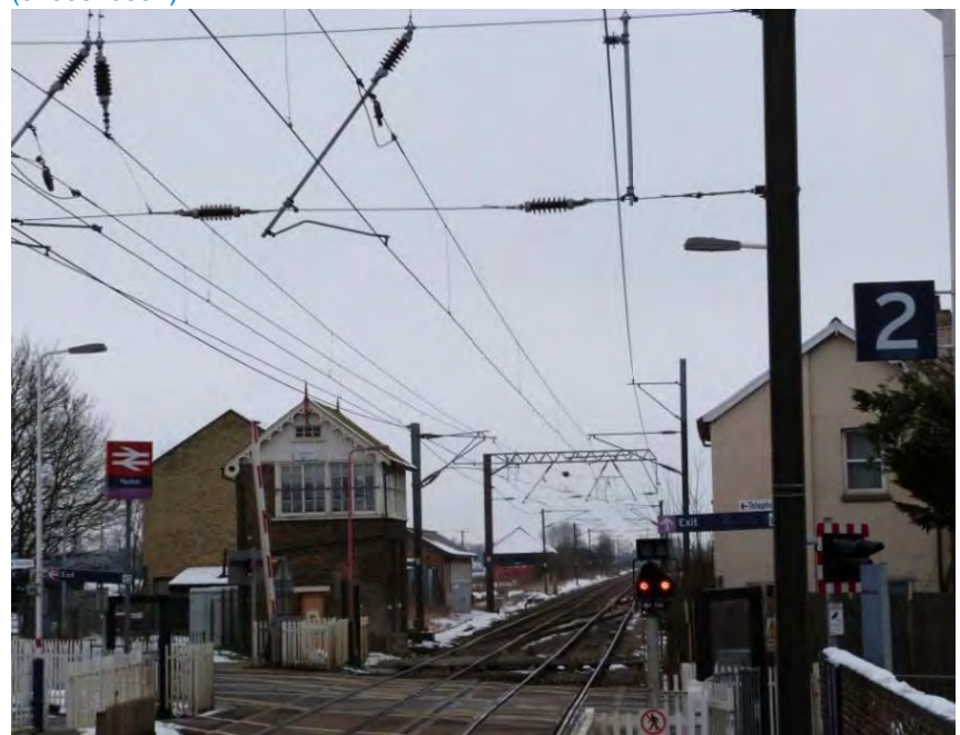
Photo 1.1: Foxton Level Crossing looking west
