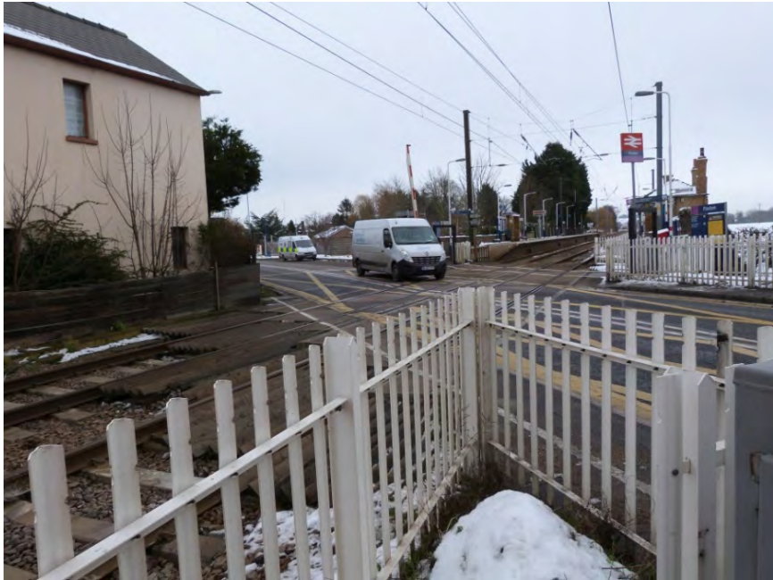
Photo 1.2: Foxton Level crossing looking north-east
